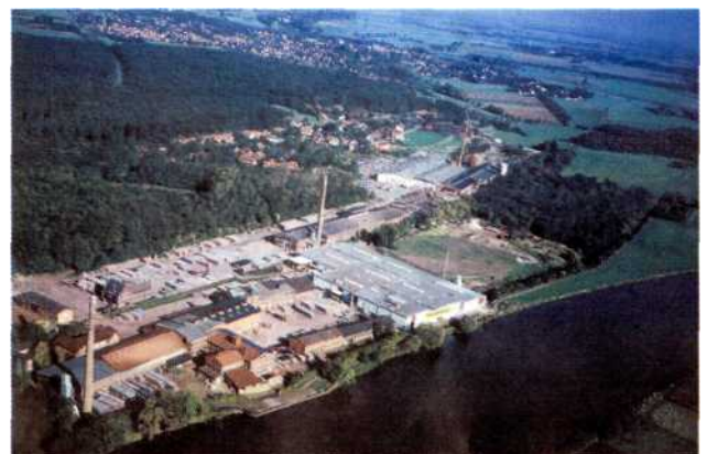
» Luftansicht des Lafarge-Werkes Petershagen » Aerial photograph of the Lafarge plant in Petershagen
